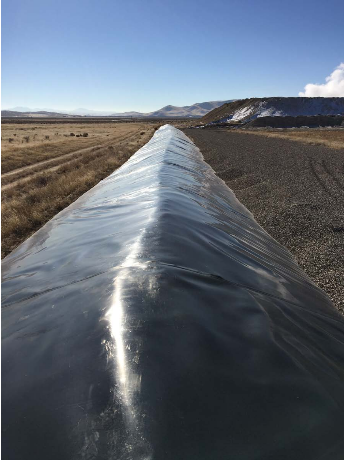
Photo 7. East Perimeter Berm, Cell 1 and 2 - View South
