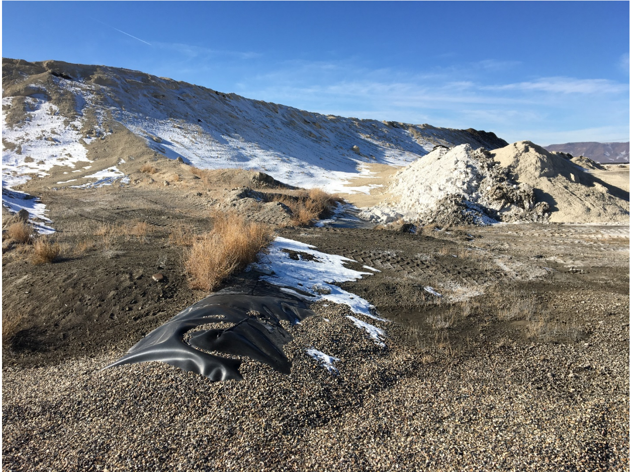
Photo 14. Transition of Deposition Cell 1 to Cell 2 - View East
