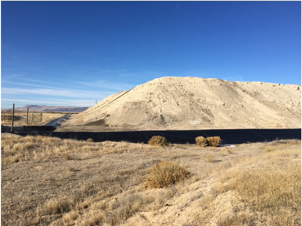
Photo 4. Southwest Corner of CCR, Cell 1 - View West
