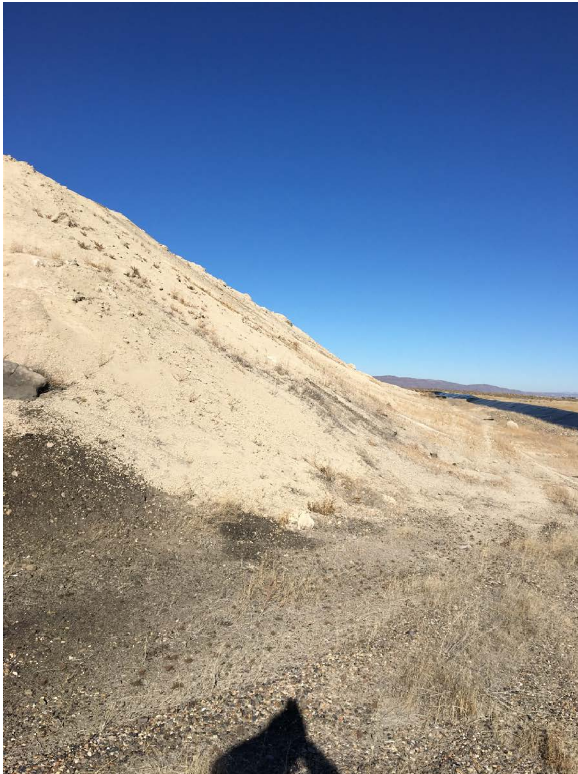
Photo 17. South Slope, Cell 1 - View East
