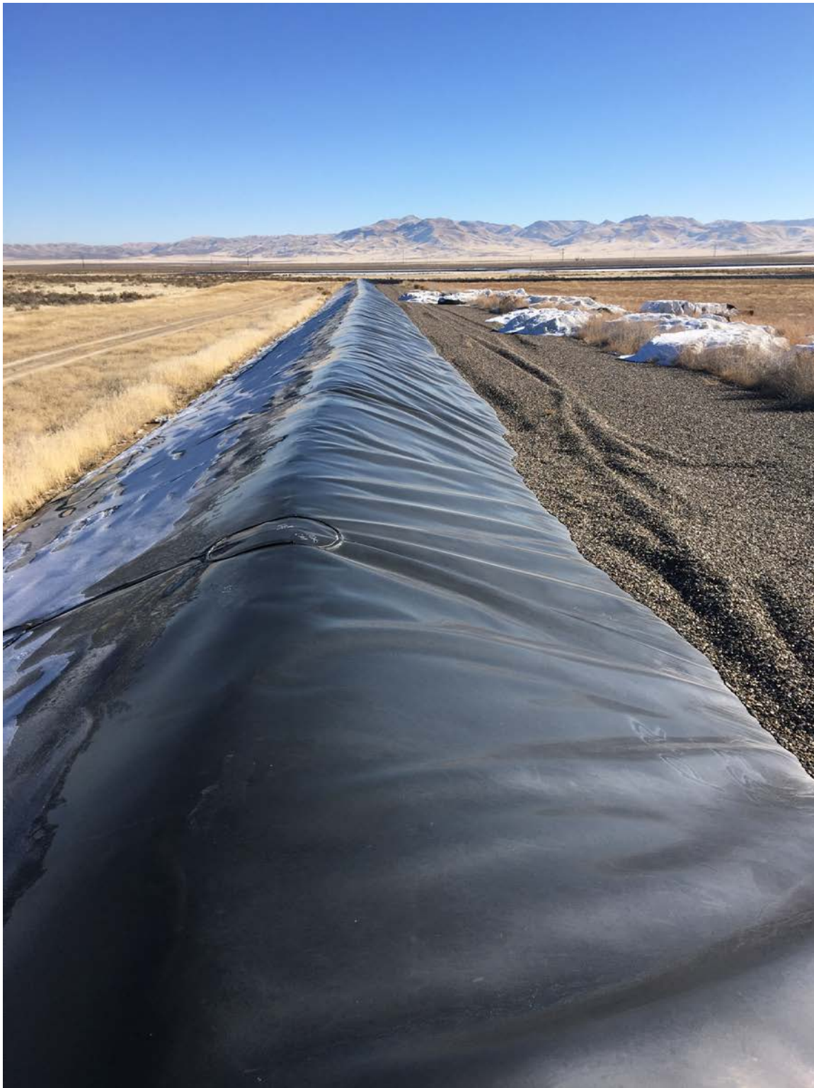
Photo 9. North Perimeter Berm, Cell 2 - View East
