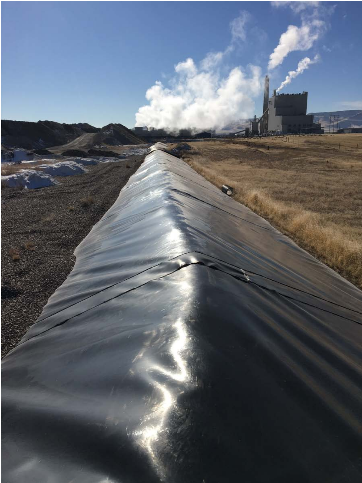
Photo 8. West Perimeter Berm, Cell 1 and 2 - View South
