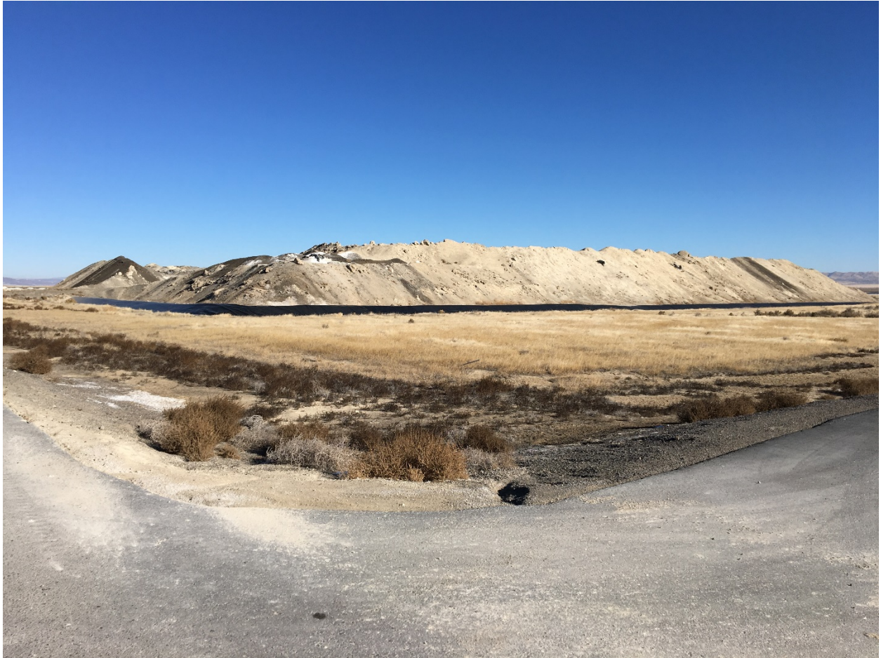
Photo 1. Southwest Corner of CCR, Cell 1 - View Northeast
