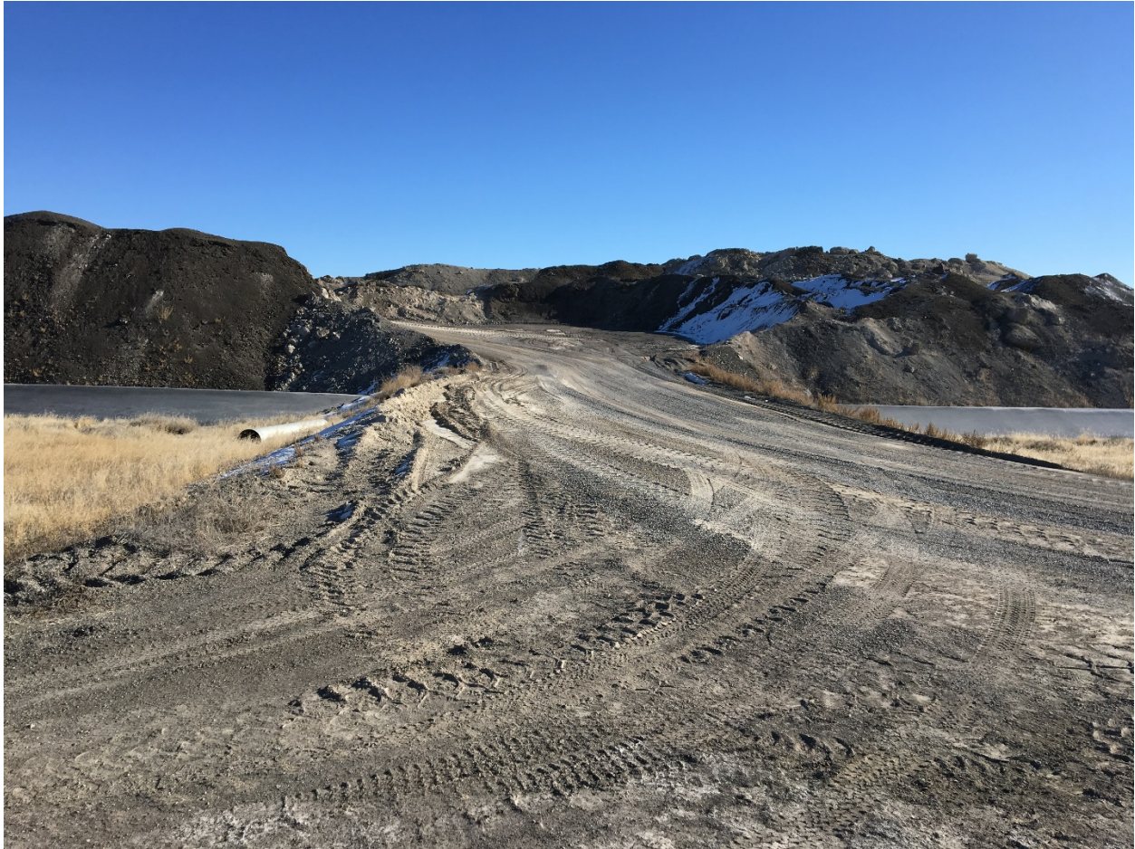
Photo 11. Access to CCR, Cell 1 - View West
