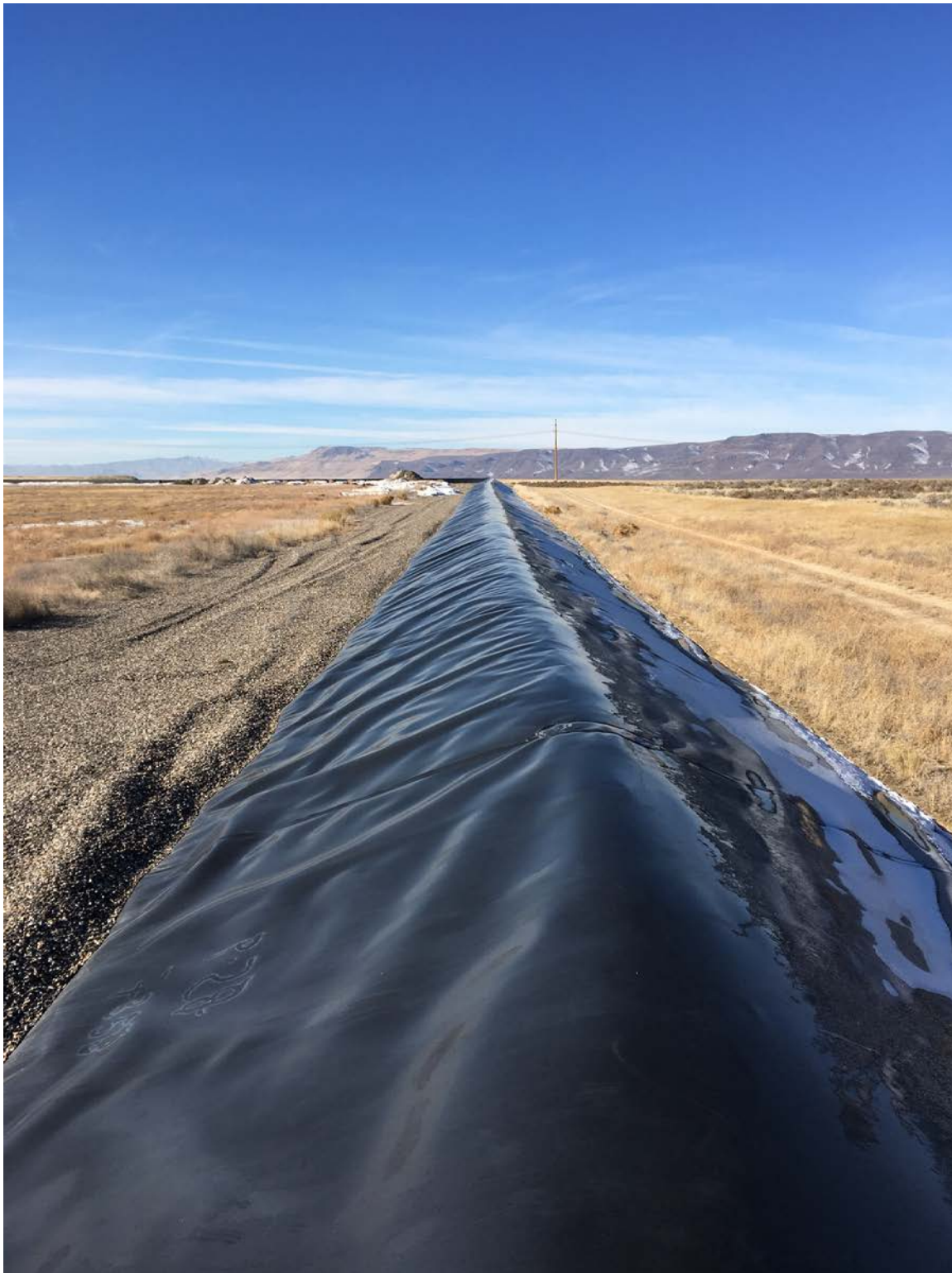
Photo 6. North Perimeter Berm, Cell 2 - View West
