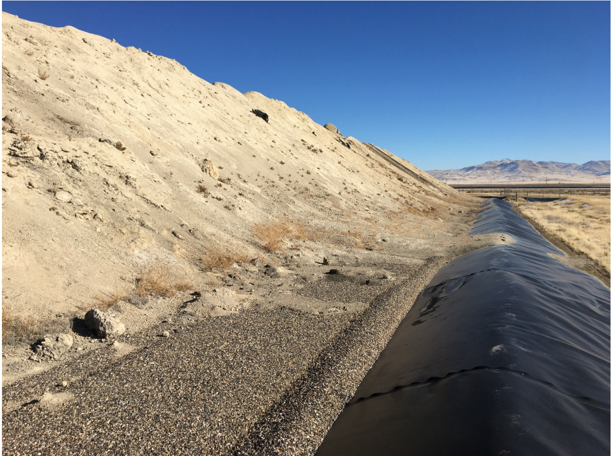
Photo 18. South Perimeter Berm, Cell 1 - View East
