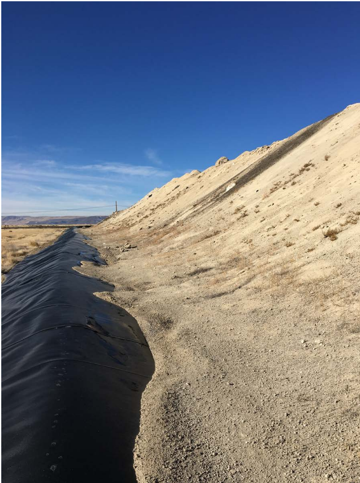
Photo 16. South Perimeter Berm, Cell 1 - View West
